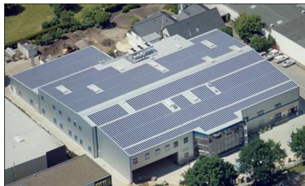
Building Integrated PV (BIPV)
